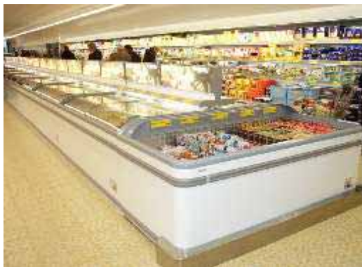
Figure 69: Self-contained high efficiency horizontal 'coffin' style freezer operating on natural refrigerants
