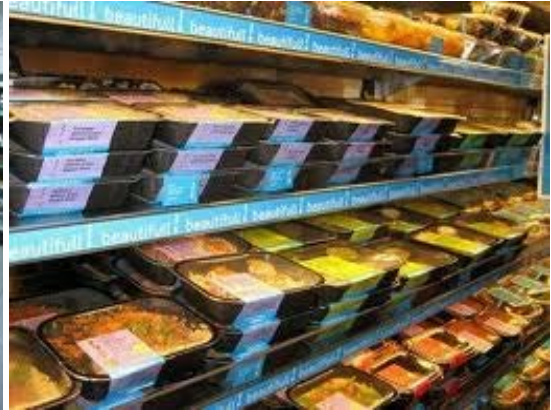
Vertical, chilled, open, multi-deck cabinet
